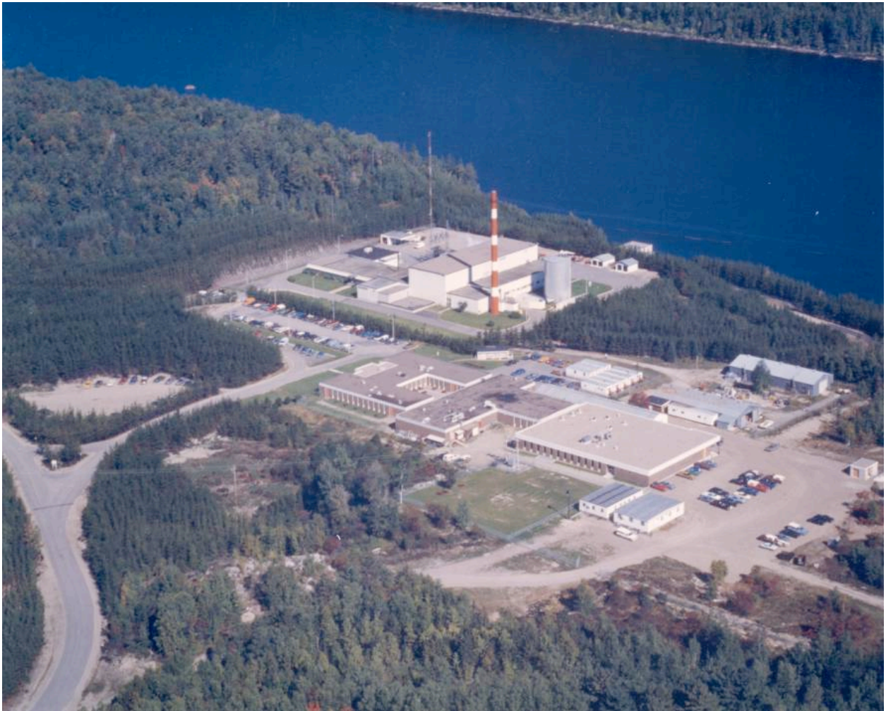
The NPD reactor seen from the air in its later years, looking north. The Ottawa River, in the background, flows from left to right. Note the large training centre. (Photo courtesy of AECL)
