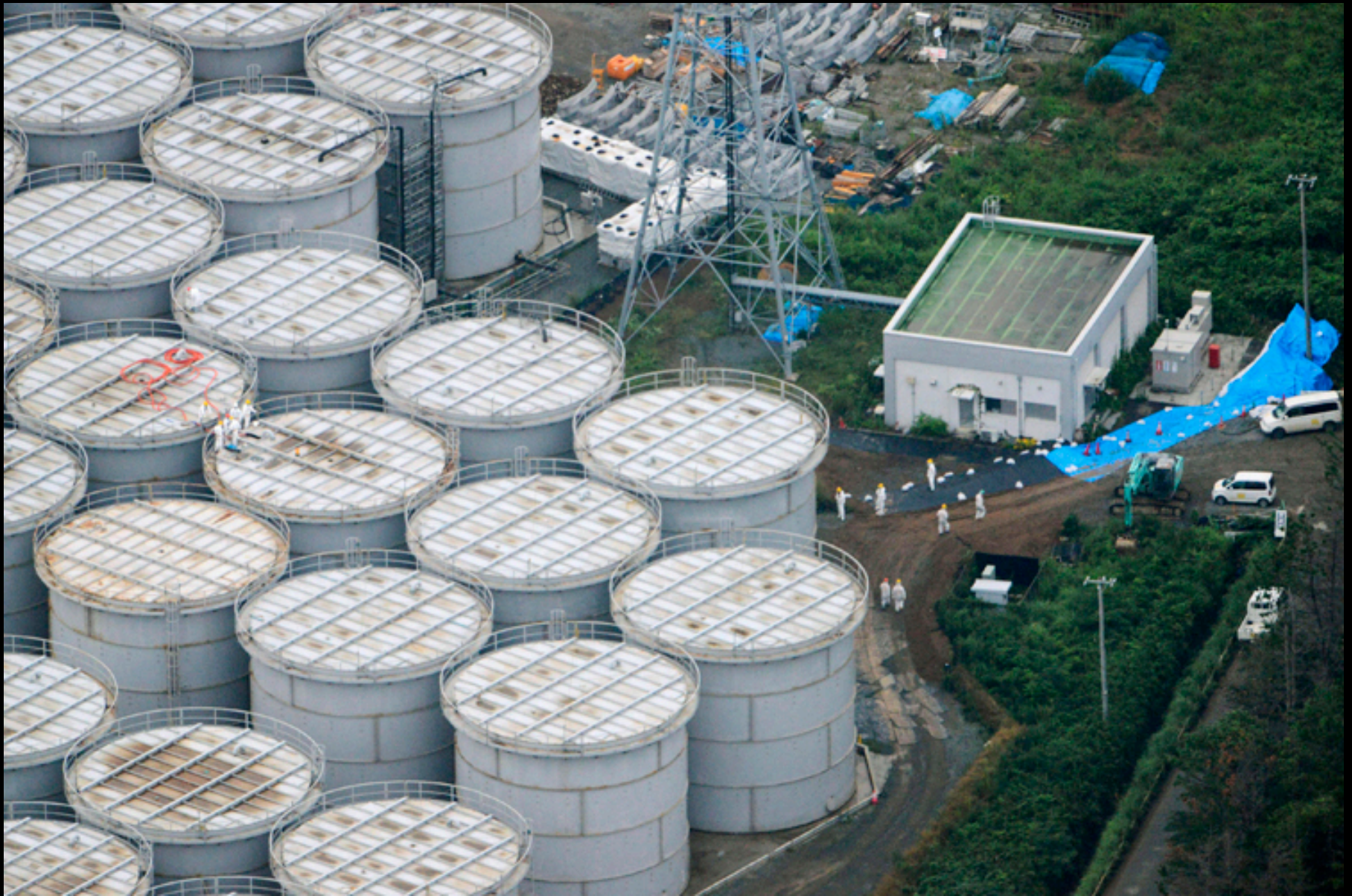
1500 tanks of highly radioactive water are already stored in above-ground areas near the plant
