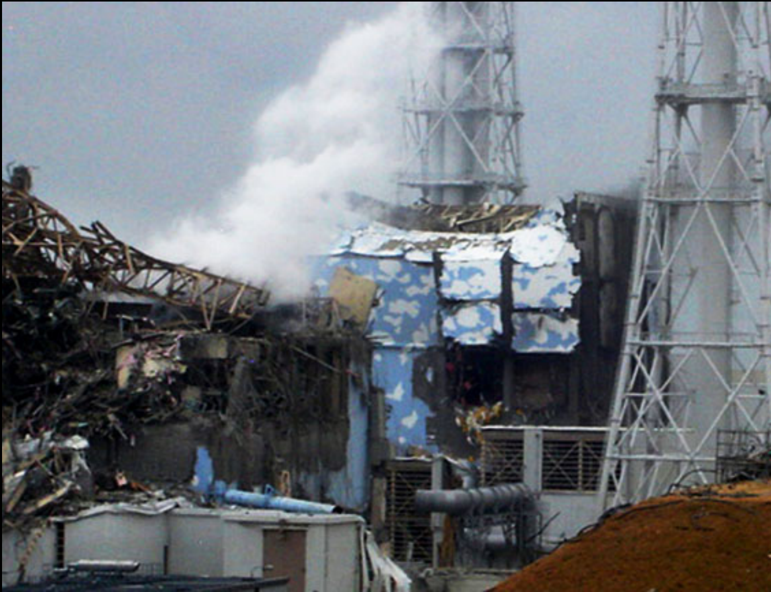
Massive damage – caused not by earthquake or tsunami, but by overheating nuclear waste
