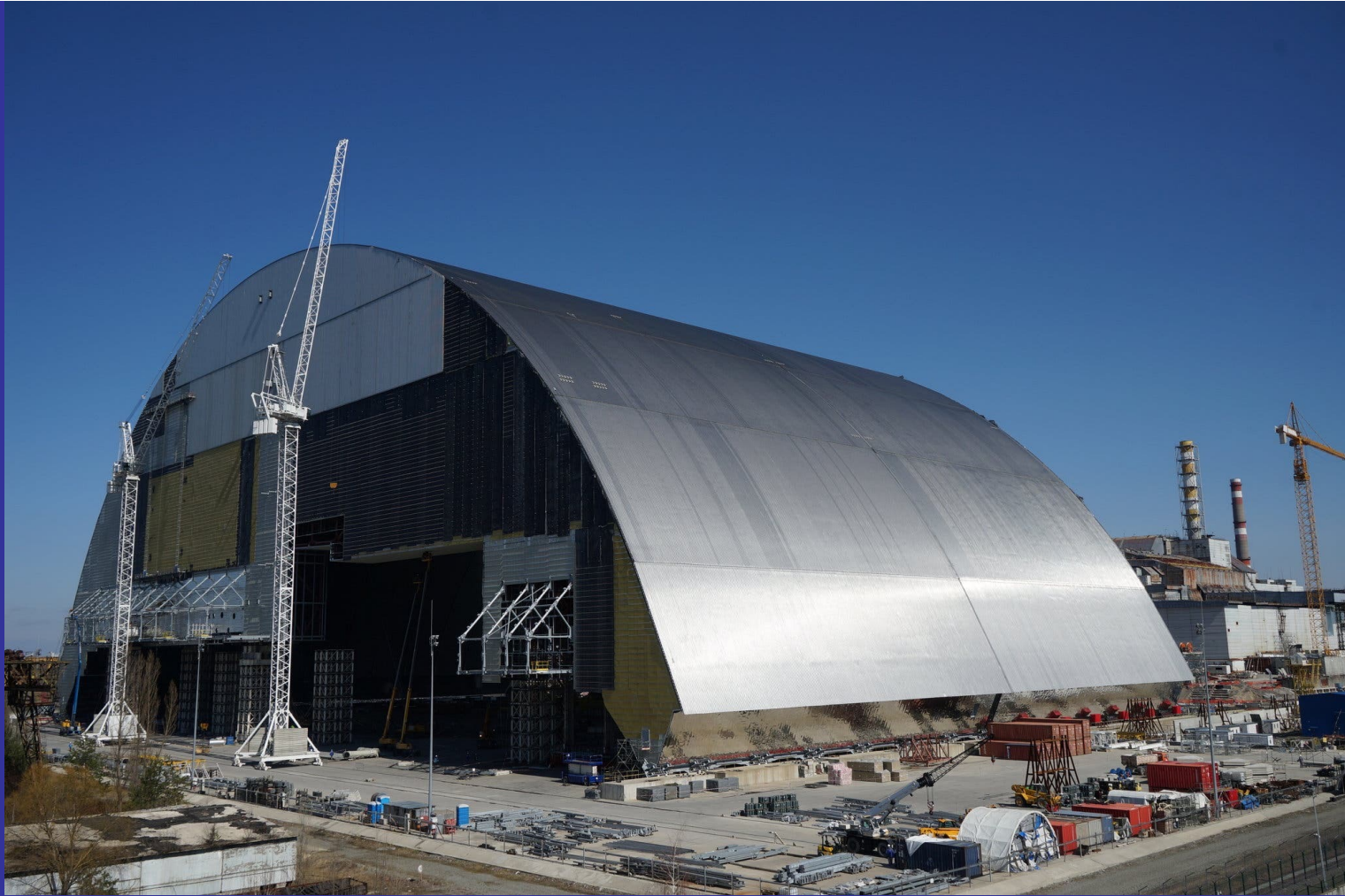
“Confinement” shelter for the crippled Chernobyl reactor installed in 2016 at a cost of US $2.3 billion
