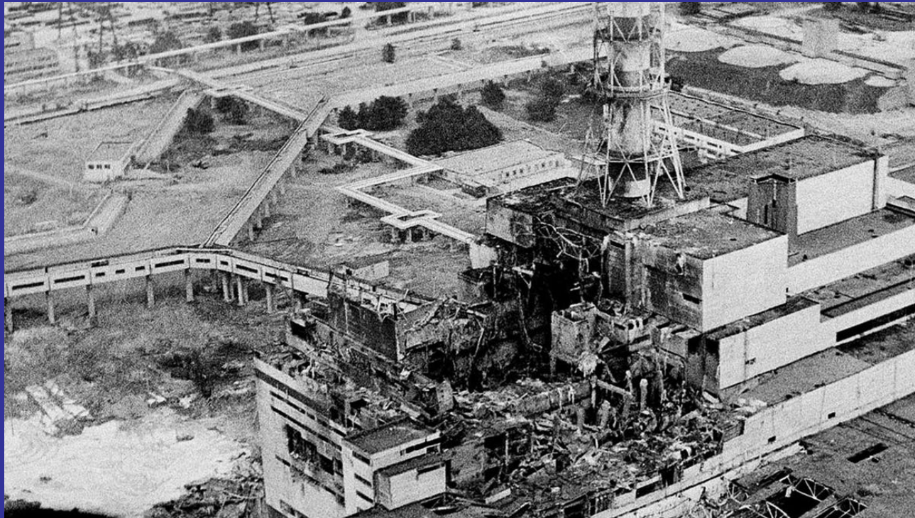
The remains of the Chernobyl reactor that exploded and melted down in 1986; explosion caused in part by “positive void coefficient”, a feature of all CANDUs
