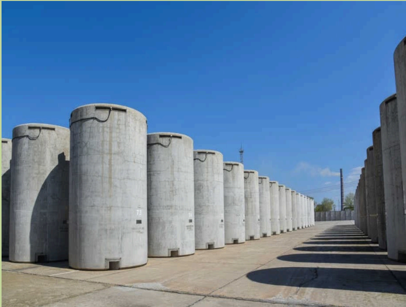
Dry storage of used nuclear fuel at Zaporizhzhia NPP – air cooled
