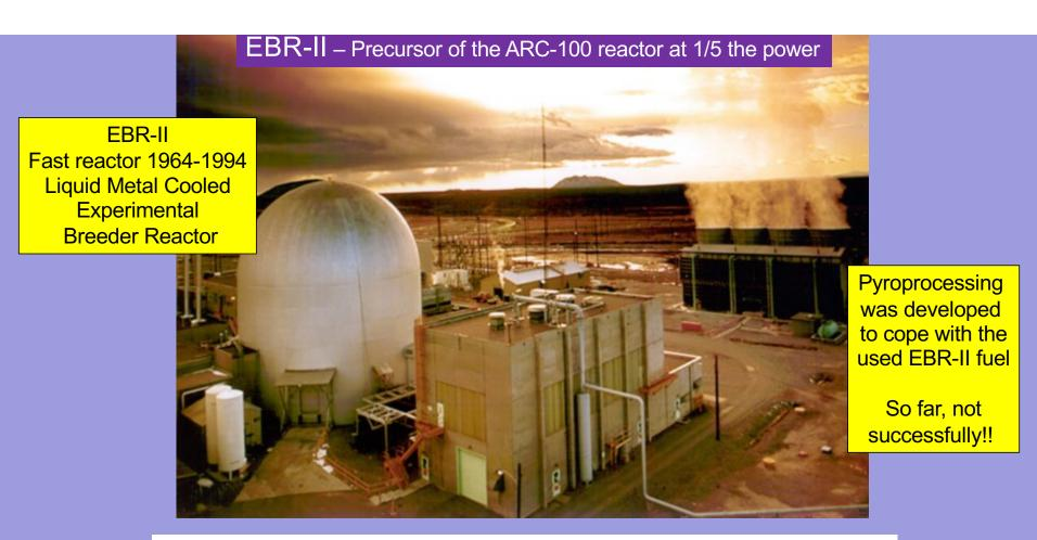
ARC-100 (100 megawatts) is supposedly modelled on EBR-II (20 megawatts) EBR-II fuel was 67 % enriched; ARC-100 fuel is 10.1, 12.1, 17.2 % enriched. A breeder reactor requires continuous reprocessing of the used nuclear fuel.
