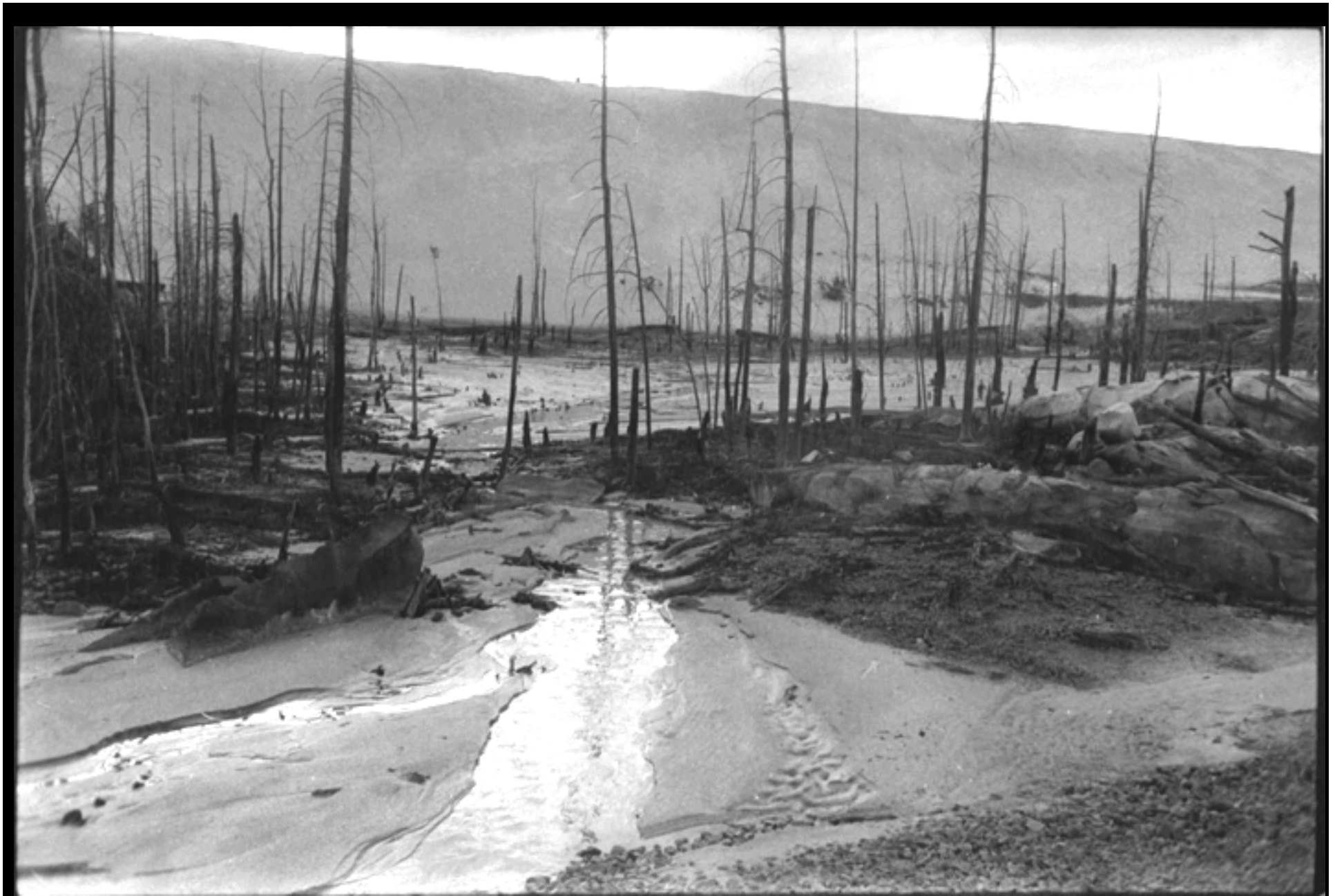
This 10-metre high wall is part of a deposit of 70 million tonnes of U tailings in Elliot Lake area.
