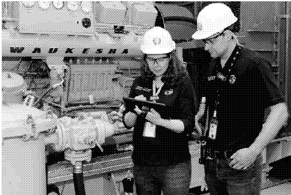
Figure 21: CNSC staff conducting an inspection at a nuclear power plant
